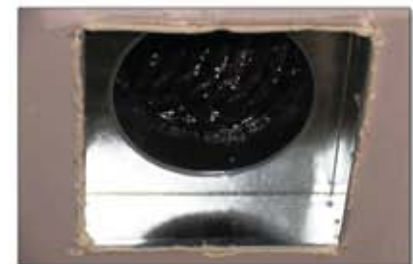
6. Additional Ceiling Air Sealing
