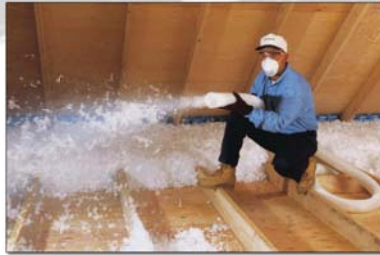
2. R42 Attic Insulation
